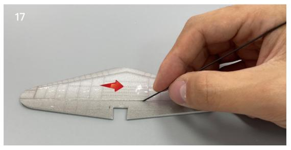
18. Use the end of a carbon fiber rod to score through the half-cut line of the rudder surface.
