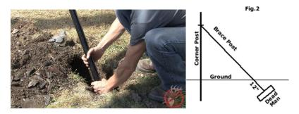
Dig a hole 1' deep where the brace post contacts the ground. Place a dead man (cinder block, large brick, or stone) in the hole perpendicular to the brace post. Wedge the brace post against the block to provide support for the vertical corner post.
