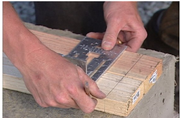
With two 2x4's side by side, mark top and sole plate in this position.
