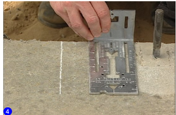
Line up tool at the 3/4 cutout with the center mark on the opposite side.
