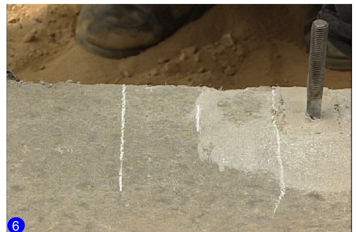
Line up tool at the 3/4 cutout with the center mark on the opposite side.
