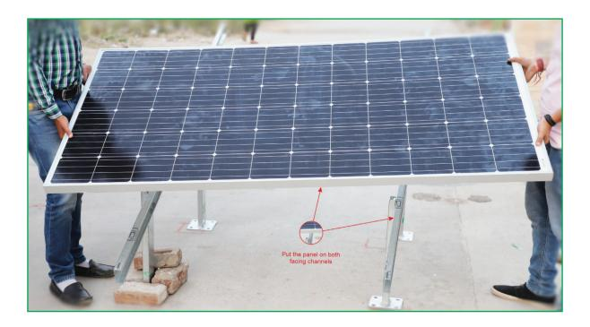
**b.** Tight Panels with Nut & Bolts- Make sure the solar panels are properly placed on the mount ing structure and tightened with the help of **nuts and bolts**. The capsule on the top of the channels should be aligned with the solar panels.
