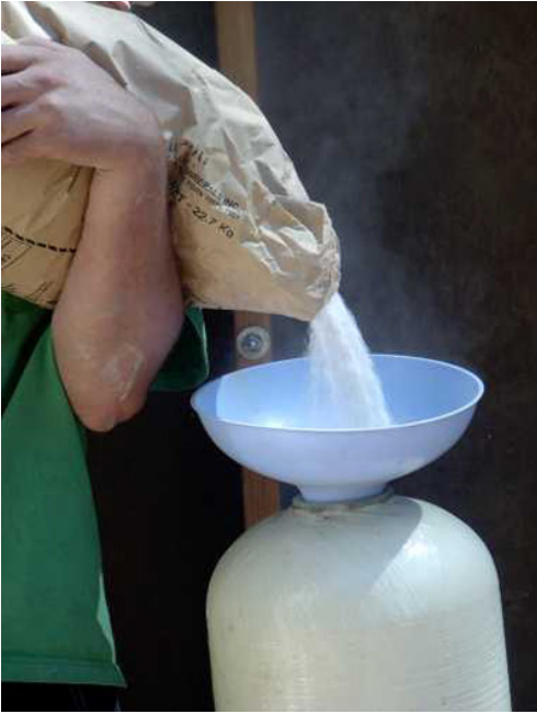
Adding media to tank.
