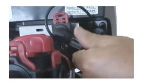
10) Connect the drain line to the control valve.
