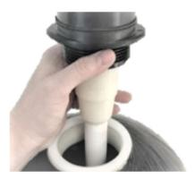
e) Install the bypass valve to the up-flow head.
