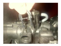
□ Push drain flow control adaptor into side of control valve and reinsert clip as shown in picture below.
