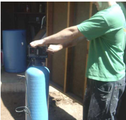
Screwing valve onto tank.
