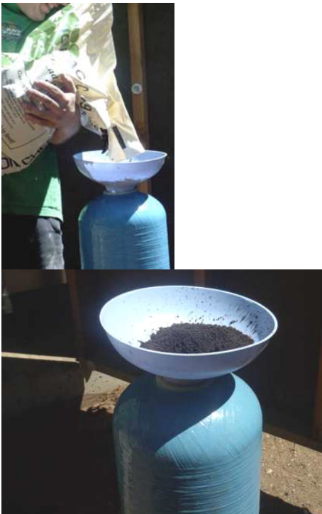
Adding media to the tank.
