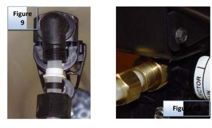
Take the other end of the tube, slide the nut/ferrule combination over it and insert sleeve into tube.
