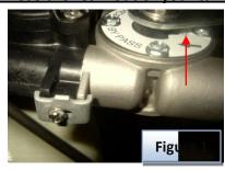
3. Use tephlon tape ONLY and wrap around the threaded end of the drain line adaptor then screw adaptor into the control valve as shown in figures 2 and 3 below. Now, snug up with a small wrench. Note: You don't have to tighten it extremely tight, it will crack the backwash assembly housing
