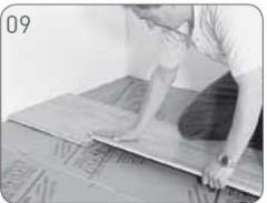
Illustration 7: The remaining boards of the first row may now be installed. Carefully align the board ends and engage the interlock by using a rubber mallet. A tight fit is an indication that the interlock has properly engaged. If the cut off at the end of the first row is longer than 40cm, it may be used as the first board of the second row, etc.
