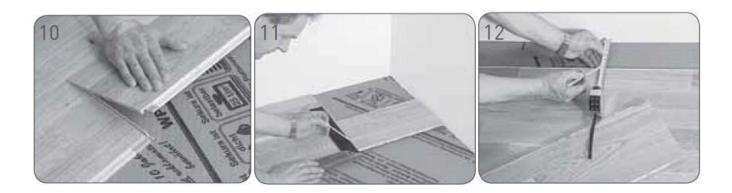
Illustration 13: For wooden or metal door frames, you are advised to establish an expansion joint of at least 3mm. Another option is to shorten the frames that the parquet floor can be pushed underneath.
