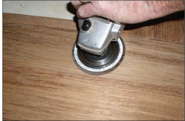
A 4-inch circular grinder creates dish out.
