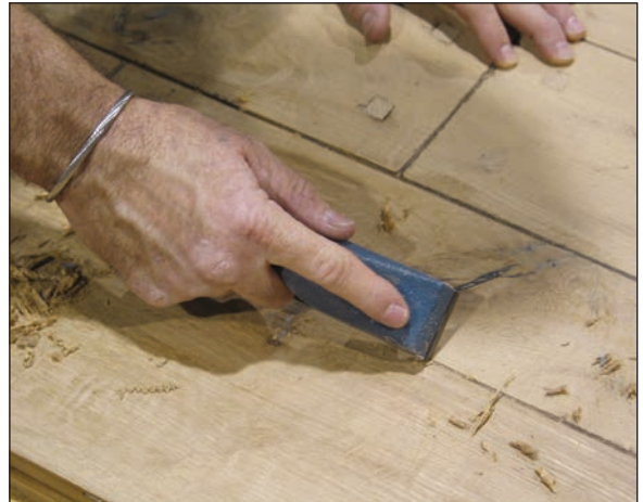
A hand-scraper pillows edges.
