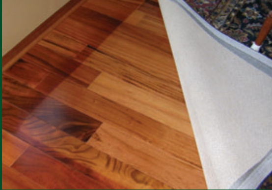
Changes in color due to differences in light exposure, such as under an area rug.
