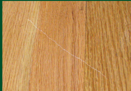
Deep scratches that go through the finish.
