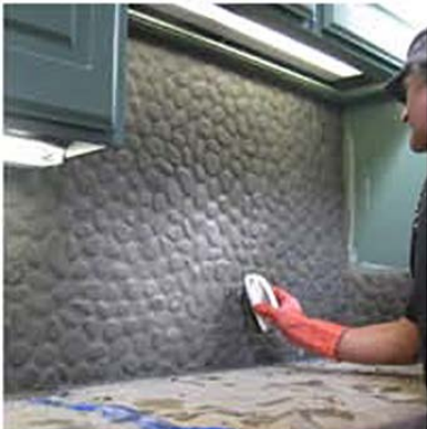
Sweep out more grout with a brush
