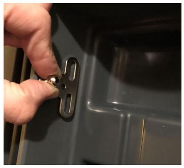
Mark the center hole and repeat the steps for mounting the lower mount
