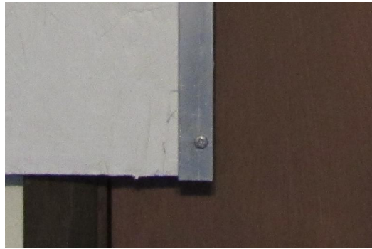
2. Place first rail with bottom screw toward opening to "stop door".
