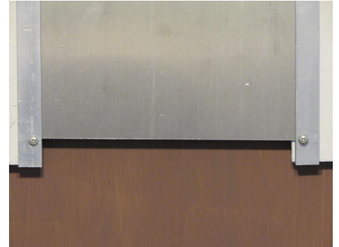
6. Check for smooth gliding: Go up and down, finish screws.
