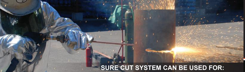
When cutting down damaged structures, there is always a danger to the operator from falling debris or material moving while being cut. With the Sure Cut System, the operator can stand on one side of the material being cut. He will first cut an access hole in the pipe, then stick the rod through the access hole and cut the pipe from the inside.
