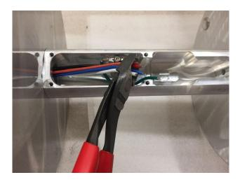
Feed the remote cable you've prepared through the connector on the Junction box cover, (Cover is in a bag in the box, along with 4 screws) slide it back on the wire, out of your way.
