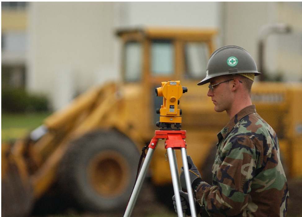
A navy surveyor using a modern theodolite
