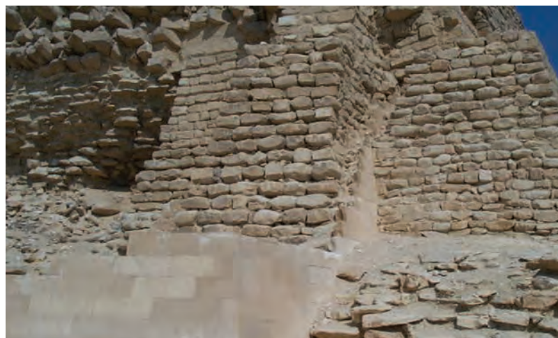
▲ The Step Pyramid started out as a single stage mastaba, then four more stages were added and then another two stages. At the northeast corner it can be seen where the final stage was added.
