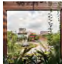
Amid the heat of Ho Chi Minh City, a green zigurat office embodies sustainable cooling strategies.
