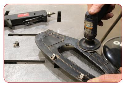
Sand down the internal plastic ribbing so it does not interfere
