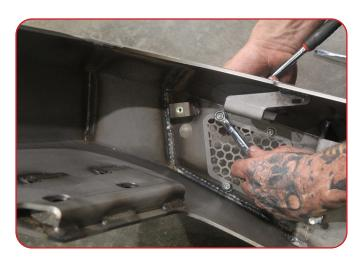
Install Covers MB1110-10, MB1110-11 & MB1110-12 with the supplied Hex Button Screws #10-24 x 3/4" long & #10-24 Nylock Nuts. Use a 1/8" hex bit & 3/8" wrench.
