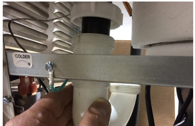
Reattach drain line to P-trap
