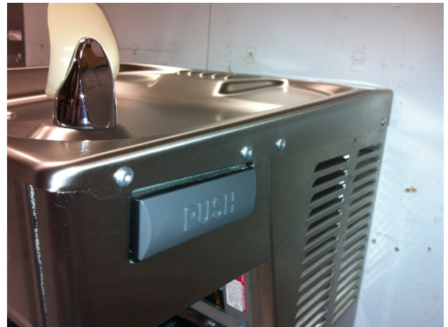
Fasten Basin Assembly in place.
