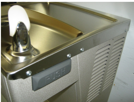
Remove Basin Fasteners
