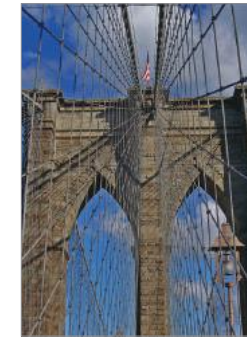
ED 303 Brooklyn Bridge Arches
