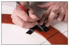
**6.** Center Dovetail Designer on overlapping gasket material and outline with pencil or awl. Cut along outline with utility knife. Top and bottom gasket materials will now have mating dovetails.
