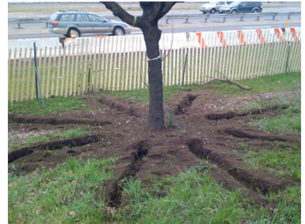
Once air-spaded, radial trenches can be filled with new or augmented soil.
