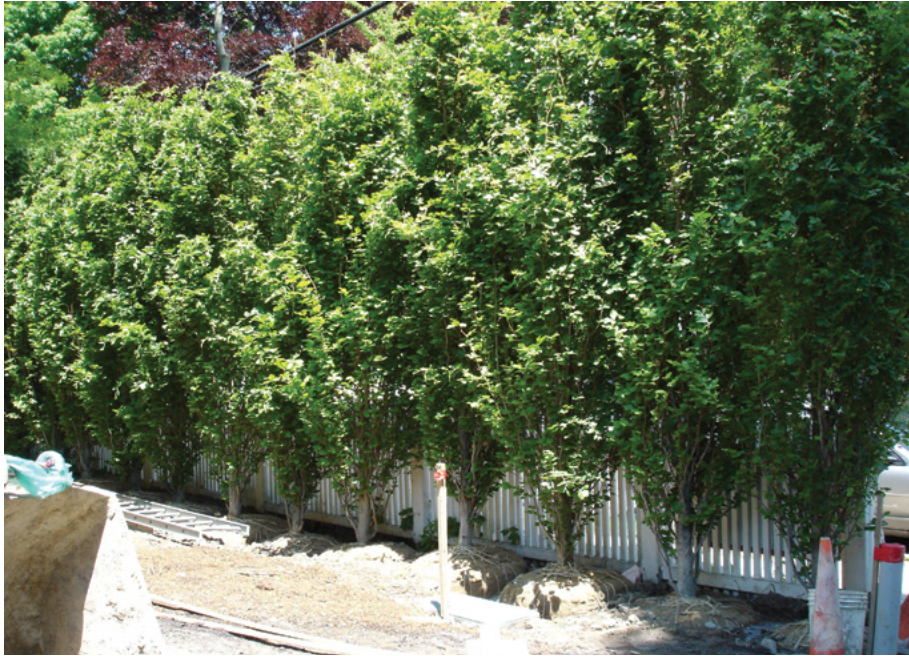
Cambridge Residence: The beech hedge shown prior to initial planting. Despite proper planting, the plants subsided, resulting in their root crown being too low, and the hedgerow soil poorly drained. Root crown excavation and drainage cores were the remedy implemented by the project arborist, and the trees have done very well ever since.
