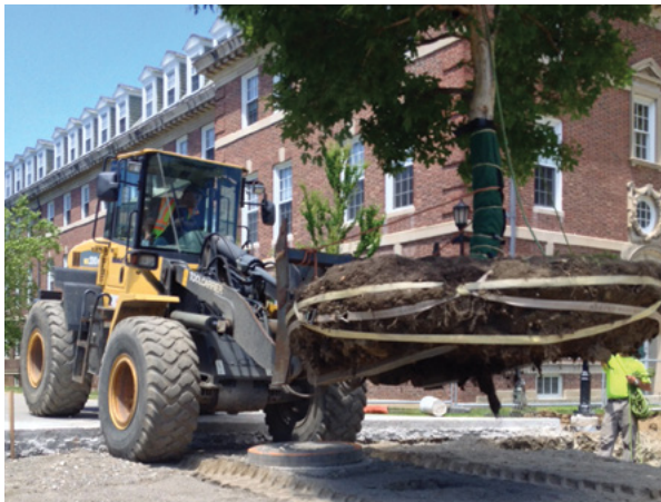
This tree at Williams College was bare rooted using an AirSpade and transplanted as part of a new quad construction project. (Image courtesy of SSA.)
