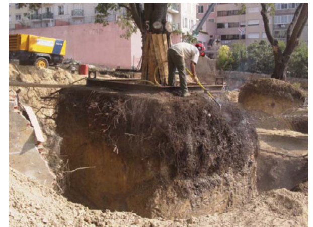
Bare rooting can allow for partial or complete soil replacement and facilitate new site construction and tree longevity.
