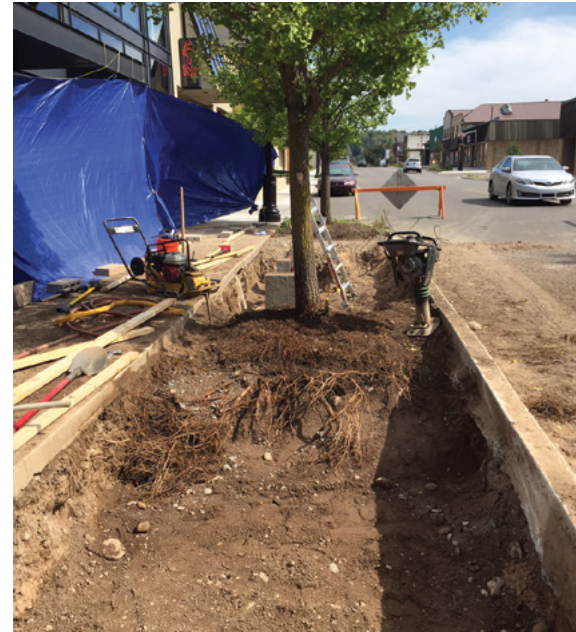
Partially bare rooted ginkgo street tree ready for new sand-based structural planting soil. (Images courtesy of Stephen Stimson Associates.)
