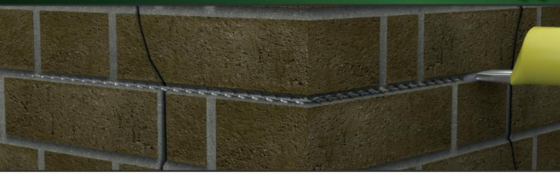
BS EN 845-1:2013 National Annex NA states that the bars need to provide an equivalent performance to the prescriptive 30mm x 5mm lateral restraint straps and the tension straps should have a declared mean tensile load capacity of at least 8kN.
