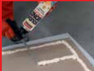
bonding of drywall panels
