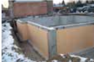
Exterior Perimeter Insulation below the soil level
