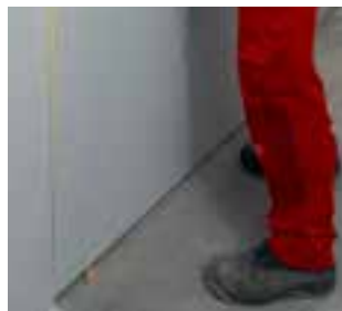
11. Only insert one spacer per panel
