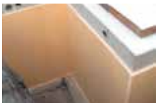
Finish the application by installing the panels in the various corners.
