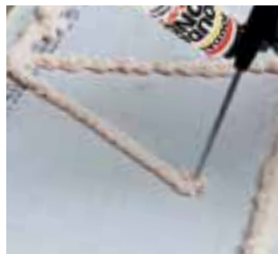
10. Apply adhesive onto the next panel with Soudabond Easy
