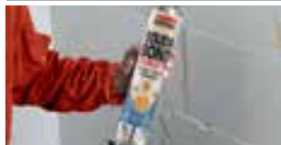
4. Shake can thoroughly at least 20-30 times
