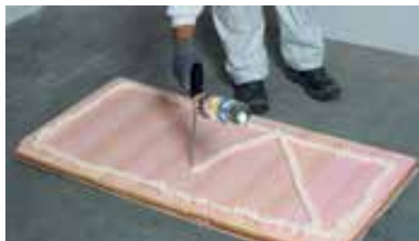
Apply Soudabond Easy onto the panel, creating closed compartments
