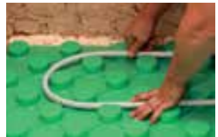
One hour after installation the subfloor heating/cooling pipes can be inserted
