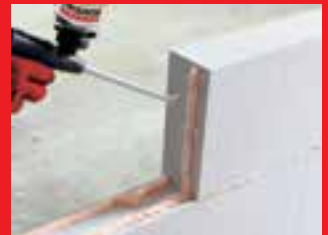
bonding of cellular concrete blocks
