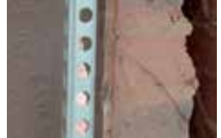
Installation of metal plastering profiles
