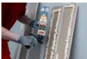
5. Apply adhesive to the panels and leave to set for 5 minutes
