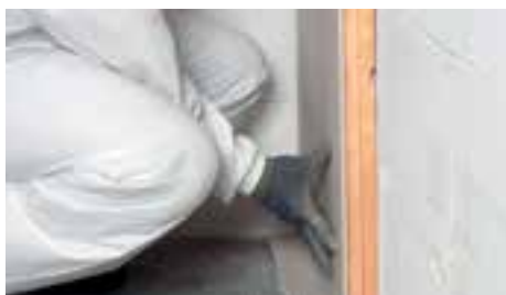
Apply pressure for ca 60 seconds. 1 hour after installation the application can be finished if necessary
