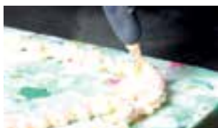
Wait for ca 5 minutes until the adhesive has built up its strength.
