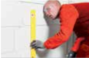
Check levelness in all directions
