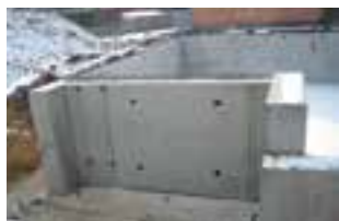
Control the substrates and remove dust, grease, etc.
