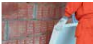
Install panel onto the substrate
