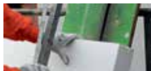
Cut insulation panels to the correct dimensions
