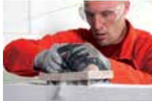
Where required scrape off material
