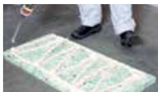
Apply Soudabond Easy onto the panel
