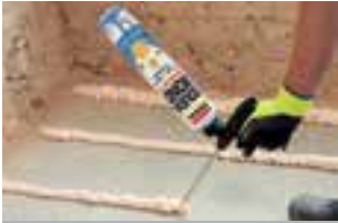
Extrude Soudabond Easy onto the substrate
