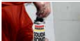
4. Remove safety cap from the adaptor
