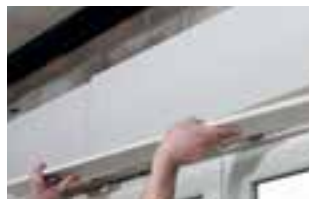
3. Check if the panels fit
