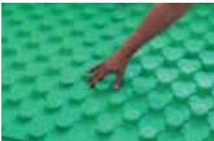
Press panels firmly into the adhesive
