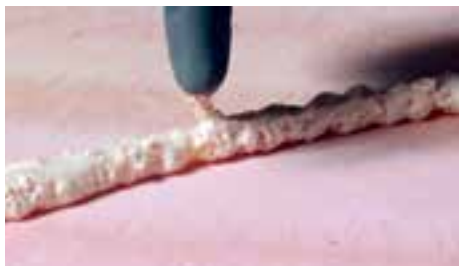
Wait ca 5 minutes (thread formation) until the adhesive has developed its strength. In this period 6-8 panels of 600x1200mm can be prepared
