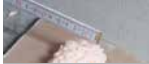
Ø 3-4cm bead – bonding on a surface with unevenness of max 1cm
