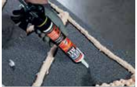
Extrude dots of Soudal Fix All High Tack or Soudal Fix All Xtreme in the empty space between the zigzag pattern
