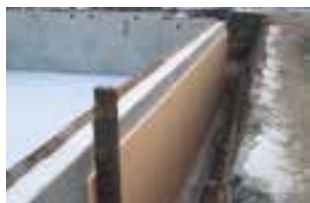
Maintain pressure on the installed panels according to the correct procedure
