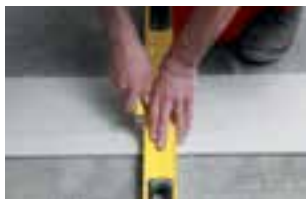
2. Cut drywall material to the required size
