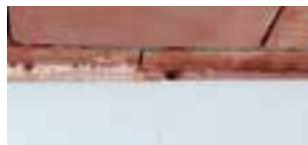
Check that there is sufficient contact with the substrate
