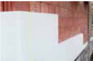
Exterior Insulation with finishing plaster layer
