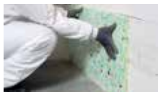
Press against the substrate and maintain pressure for ca 60 seconds
