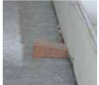
6. Press on completely, ensure that the panel is 100% vertical on the other side, if necessary place wedge
