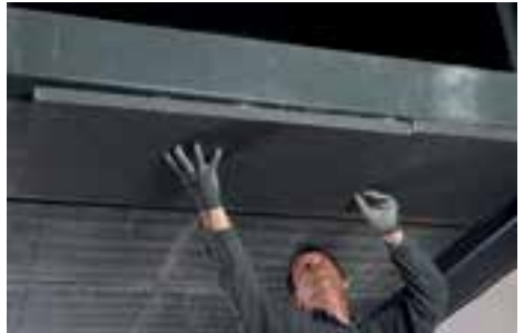
Press strongly into substrate
