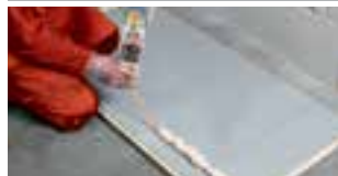
6. Apply with the valve pointed downwards
