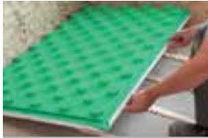
Insert studded panel into the adhesive beads
