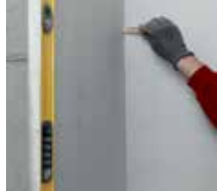
5. Control that the panel is 100% vertically even, if necessary place wedge
