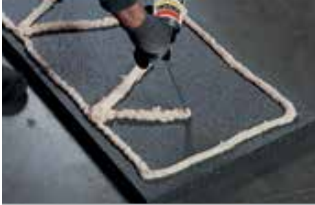
Extrude Soudabond Easy onto the insulation panel
