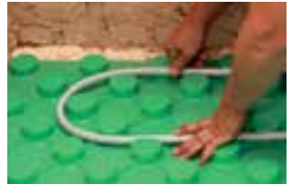
Insulation with subfloor heating
