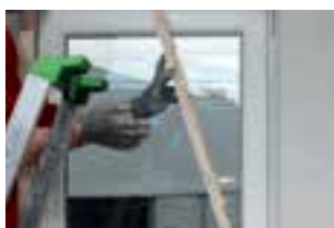
8. Install side reveal n°2 and support lathes
