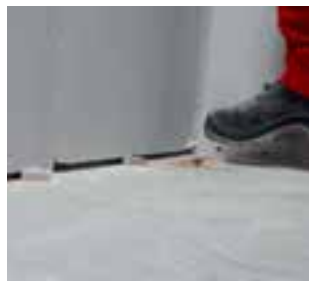
12. Insert the panel into its space ca 5 minutes after applying the adhesive and check on the horizontal, vertical and diagonal evenness
