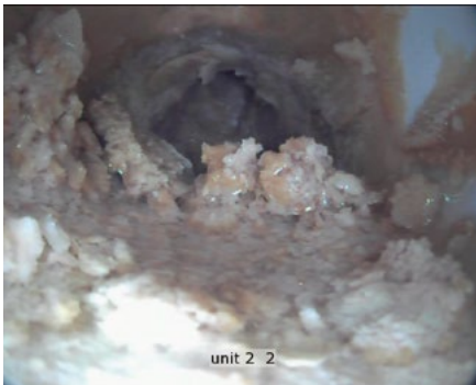
Typical problems caused by lime deposits
