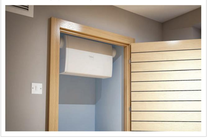
PIV systems are proven to be effective units in significantly reducing radon gas levels in affected areas.
