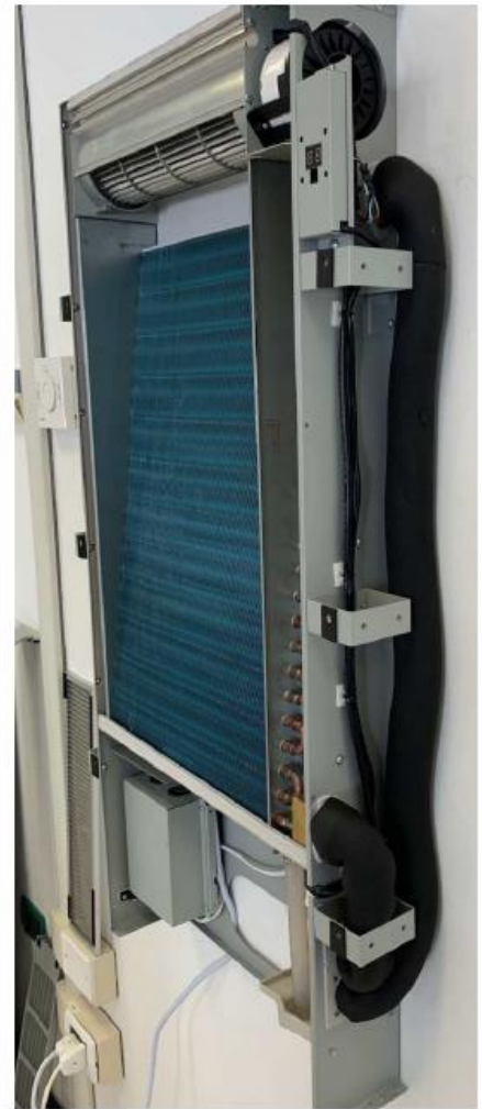
PUT INSULATION IN ALL THE EXTERNAL PIPE
