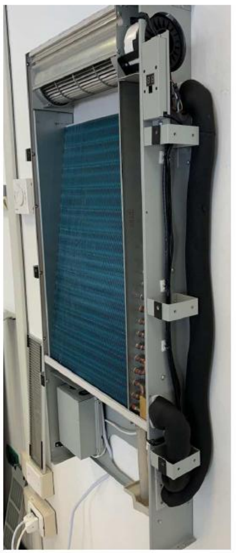
PUT INSULATION IN ALL THE EXTERNAL PIPE
