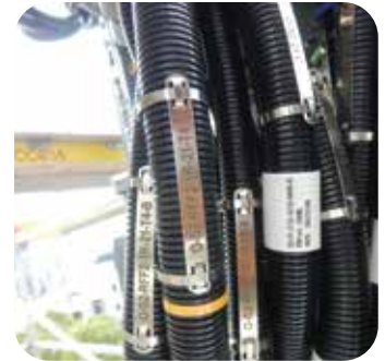
316 grade SS tags installed with 316 or 304 grade SS cable ties.
