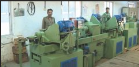
Automatic Strip grinding line from Solingen
