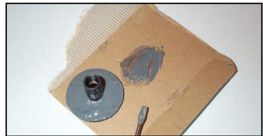
Figure 24 - Coat the topside washer of two of the rivnuts
