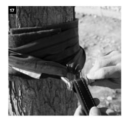
Next, dismantle the anchor on this side by unscrewing the shackle pin to remove the ratchet and round slings then the tree protection. Move to the opposite tree and repeat steps above.
