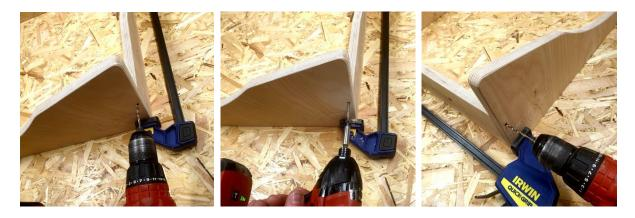
Stage 5: Drill a 4 mm x 55 mm deep hole through the bottom marker point in the side panel and fix with a 5 x 50 TX25 Screw. Turn the construction around and repeat the same in the opposing bottom hole.
