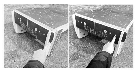
The plates attach to the hinged part of the Tabletop with M10 x 40 mm Bolts through the locations / holes shown below. Tighten these bolts fully before moving onto the next stage.
