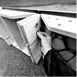
Alternatively, roll the Tabletops over so they are upside down. Tighten the bolts on the joining plates
