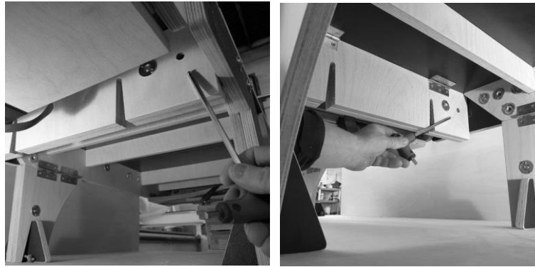
BOLTING TWO TABLETOP END PLATES TOGETHER
