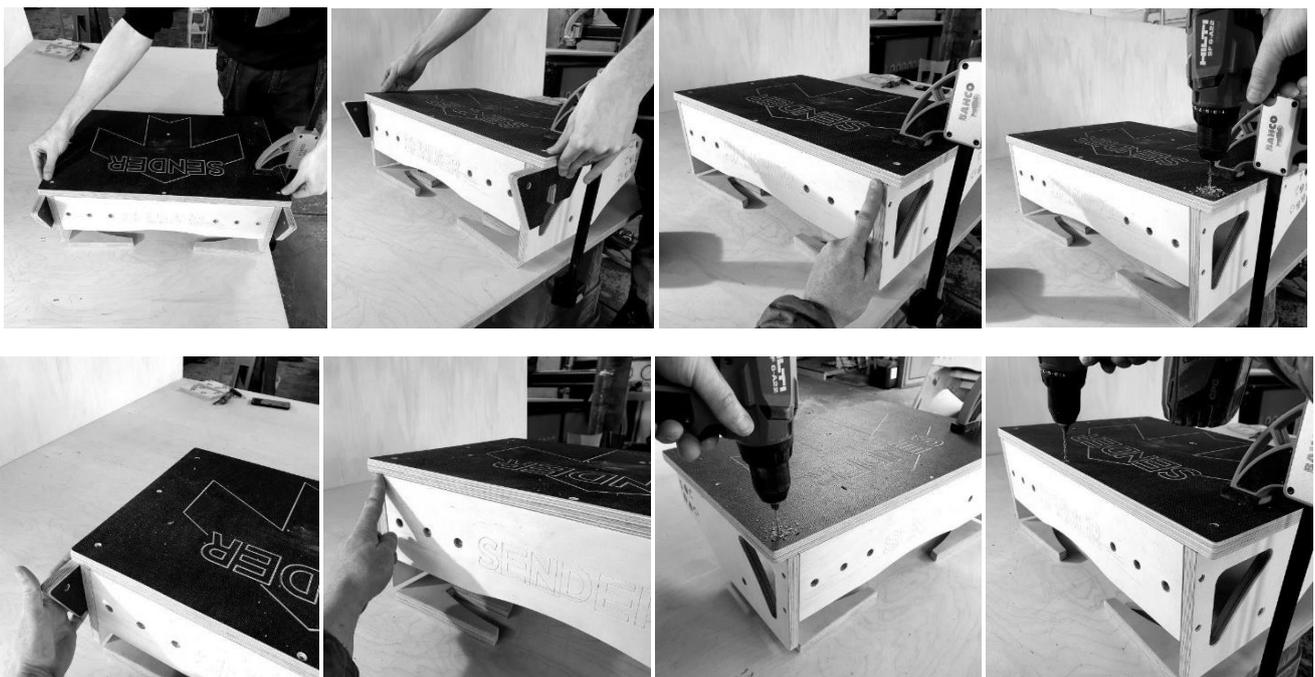
The BACK PLATE is also secured in the middle at the edge of the surface. YOU MUST DRILL AND SECURE AT A SLIGHT ANGLE! To prevent the plywood bulging or the screw appearing on the front or back of the BACK PLATE! There are 3 additional fixing points on the surface. One on either edge and one in the centre.
