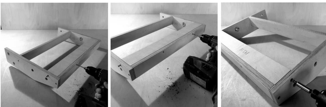
Complete the process of fixing PG V by drilling through the side panels and fixings with TX25 Screws as shown below. **THE EXPERT PROGRESSION RAMP HAS 2 x TX25 Screws EACH SIDE OF BATON PG V!**
