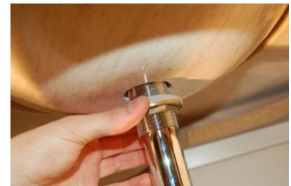
Thoroughly tighten the nut onto the threaded pipe of the drain, securing the sink and drain in place.
