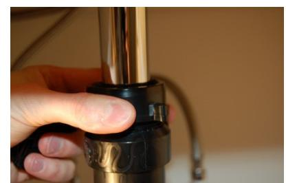
Tighten the female trap adapter attached to your drainage pipe until it securely grips the drains tailpipe.
