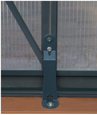
Internal ground anchoring system
