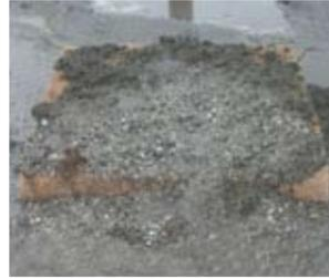
Inlet Filter will collect a lot of sediment. Clean Inlet Filter while mounted on the grate, even if ponded water surrounds the inlet. This unique feature insures all water entering the grate is filtered. Sweep sides and top of Inlet Filter to remove sediment and debris after each rain event.
