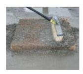
2. Remove sediment from the top of the filter by sweeping off of Inlet Filter.
