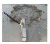
**1. Remove sediment** from the sides of the filter by sweeping away from Inlet Filter.
