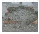
Inlet Filter will collect a lot of sediment. Clean Inlet Filter while mounted on the grate, even if ponded water surrounds the inlet. This unique feature insures all water entering the grate is filtered. Sweep sides and top of Inlet Filter to remove sediment and debris after each rain event.
