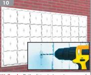
Wall only: Drill a fixing hole at the centre of each and every cell to suit your desired shape and area, then remove the Templates and install rawlpluas.
