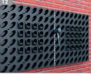
Assemble next panel as per steps 1-8, connect to existing fixed panel and secure as per step 11. Repeat the process until the desired shape and area is covered
