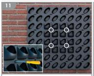
Position your G-WALL and using suitable screws, secure the four central cells through their spigots to the corresponding fixing holes
