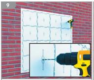
Flatten G-WALL Template & position on your wall or suitable structure. **Wall only:** Drill a fixing hole at the centre of each cell (16), then remove the Template and install rawlplugs.
