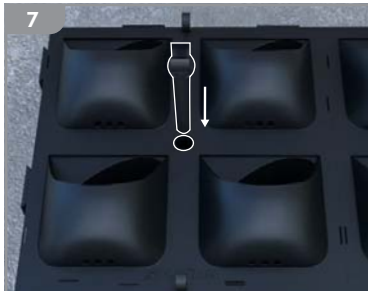
Insert the fixing spigot into the hole in the centre of the Fascia and G-WALL Cell, ensuring that it clicks into place.
