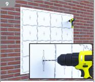
Flatten G-WALL Template & position on your wall or suitable structure. Wall only: Drill a fixing hole at the centre of each cell (16), then
