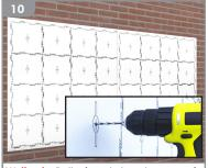
Wall only: Drill a fixing hole at the centre of each and every cell to suit your desired shape and area, then remove the Templates and install rawlplugs.
