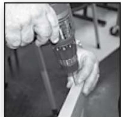
**6.) Place silicone on threads of #10 x 3/4" screws.**
