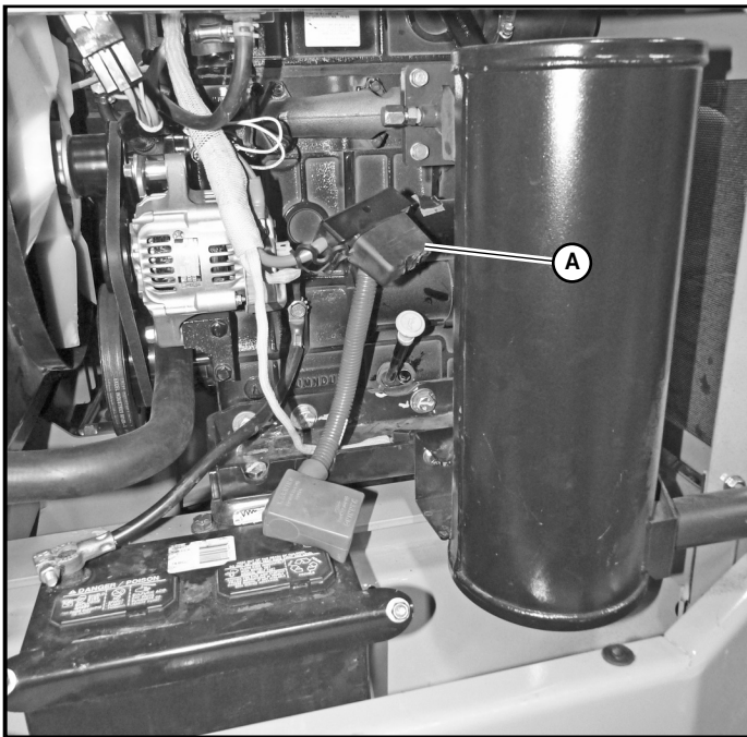
A. 50 Amp fuse housing
